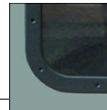
Detail of ABS Window Frame
